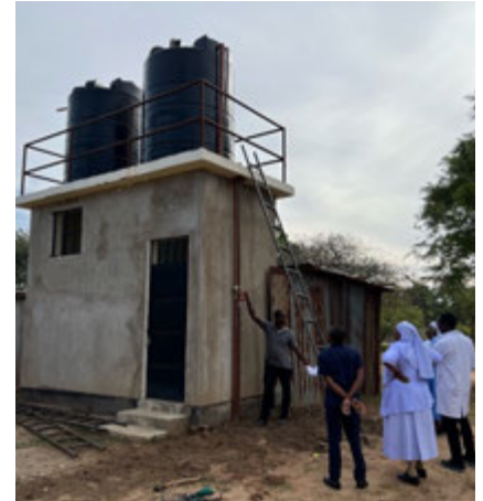
2 x 2000 l Wassertanks, neu
